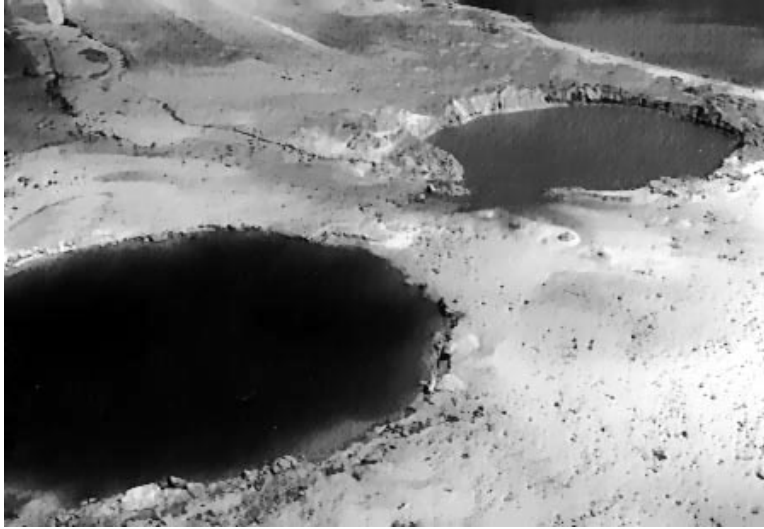
Fig. 20: Twin craters created by the Cactus and Lacrosse tests on the Runit island. The left crater was used to isolate contaminated soil, now designated as the Nuclear Dome.
