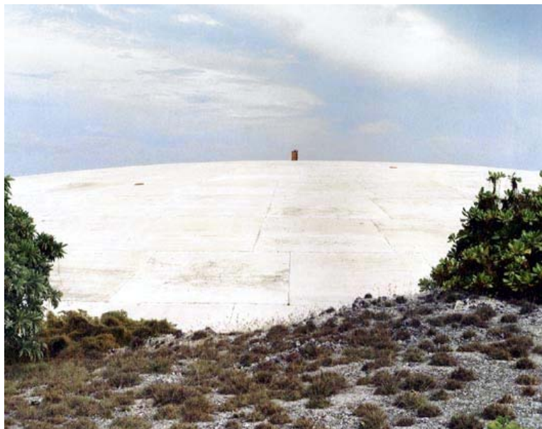
Fig. 19: Concrete dome 18 inches in thickness entombs 111,000 cubic yards of contaminated soil and debris on Runit Island. As a prank, a red painted barrel on its top makes it visible from aircraft.
