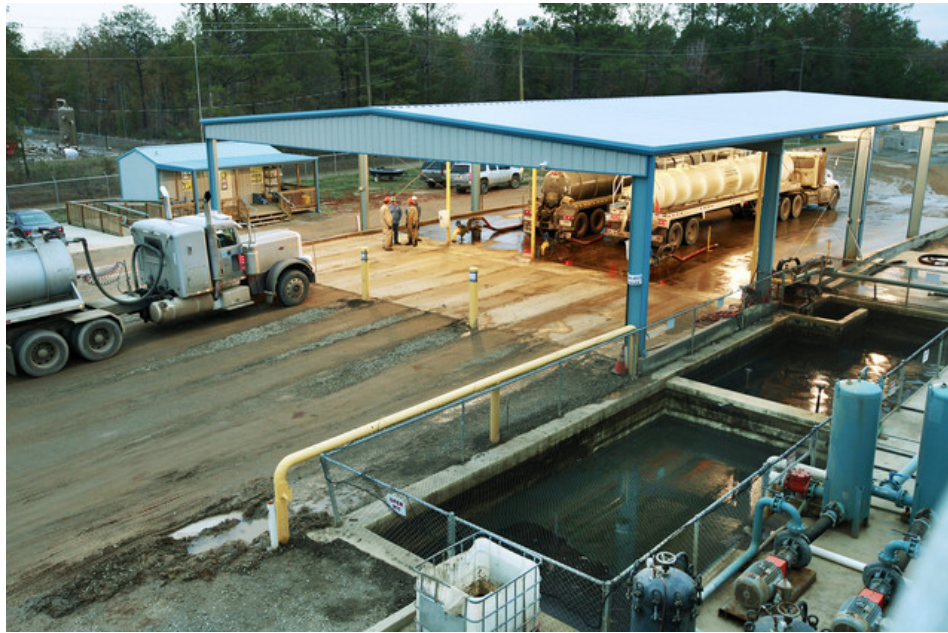
Figure 19. Water treatment plant for the separation of oil, sediment and antifreeze, Camptown, Pennsylvania, Marcellus formation. Source: Bloomberg.
