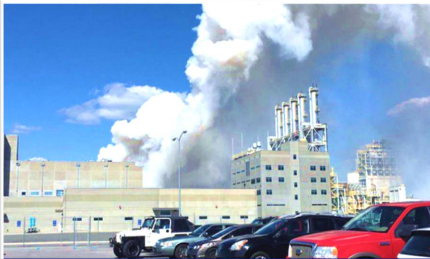
Faulty piston caused explosion at Wacker's U.S. polysilicon plant
