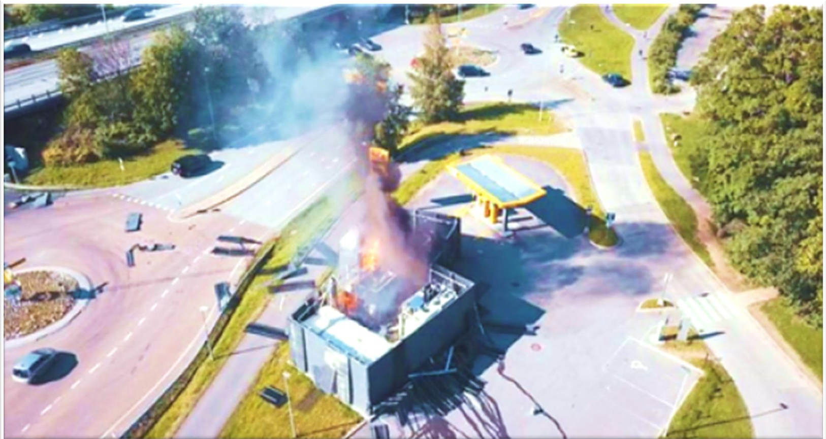
Hydrogen Refueling Station in Norway Exploded
