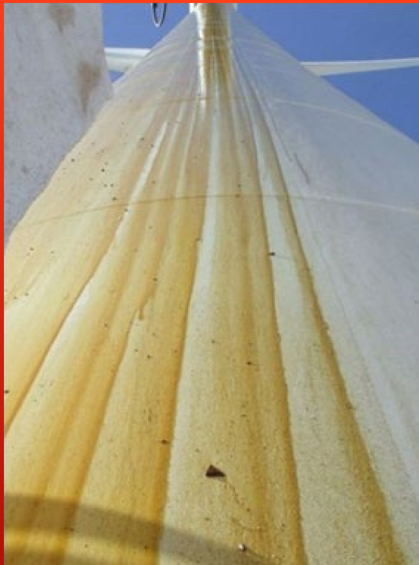
Wind Turbine oil spill
