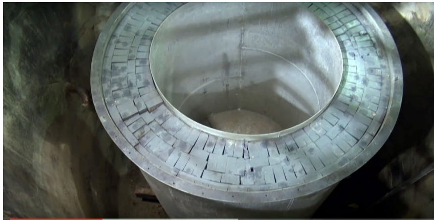
Figure 4. Graphite blocks reflector surrounding an unfinished reactor core.
