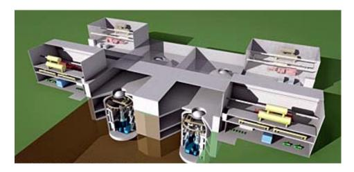
Figure 2. Compact Underground Reactor in a 4 units 500 MWe configuration of 125 MWe each. Source: Babcock & Wilcox.
