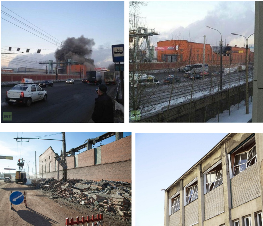
Figure 20. Blast wave and debris effects of Chelyabinsk meteorite on a zinc factory, power lines and window frames February 15, 2013. Source: RiaNovosti.
