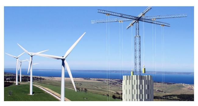
Figure 1. Wind turbines electricity stored then retrieved from a gravitational potential energy storage tower.
