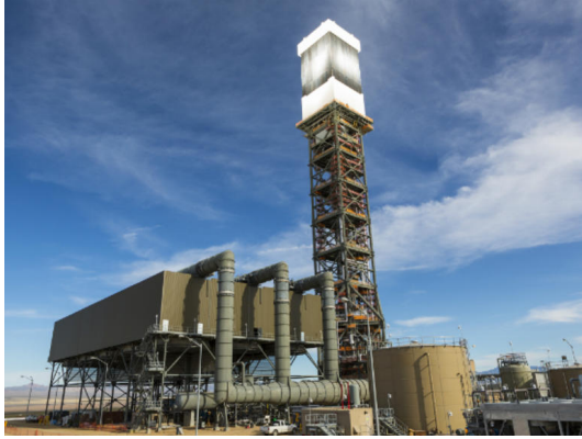
Figure 48. Boilers of the Ivanpah plant. Owned by NRG Energy, Google and BrightSource Energy. Plant does not use energy storage, but steam is used for the secondary recovery of oil by the Chevron oil Company.
