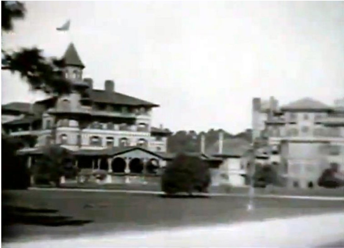
Figure 50. Jekyll Island Club retreat, Georgia, USA.
