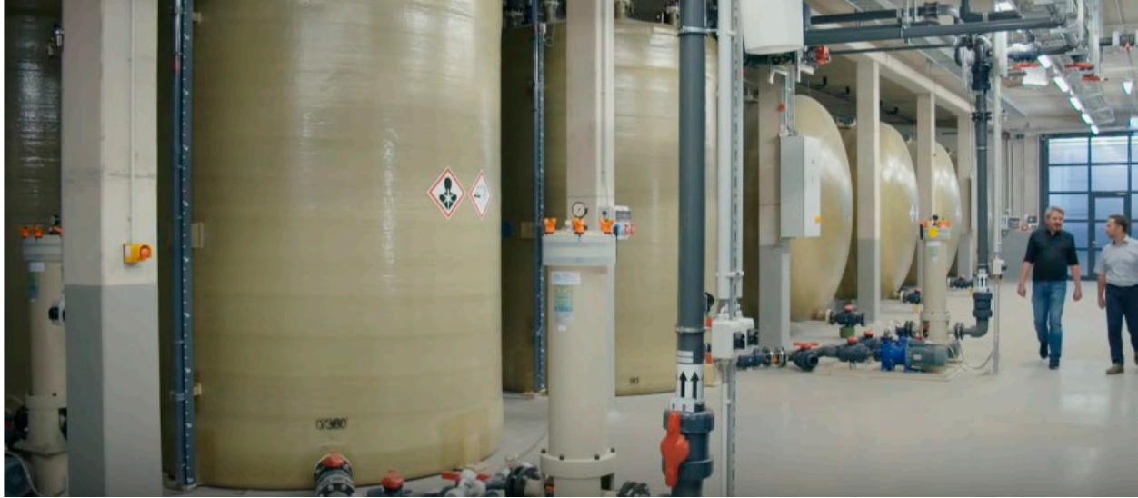
Figure 19. Large scale Redox flow batteries can store energy from consumer-owned DC current-producing wind turbines over long time periods without being connected to the grid.
